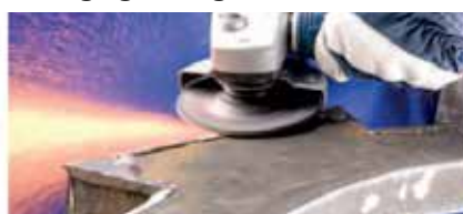
Rough grinding & weld removal
