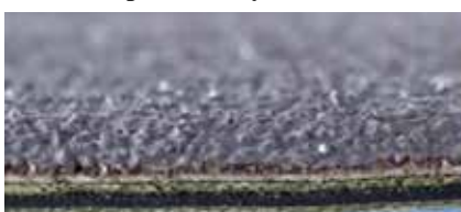
Close up of the layer structure
