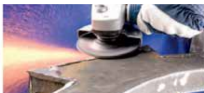
Rough grinding & weld removal
