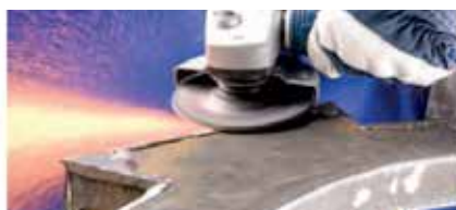
Rough grinding & weld removal
