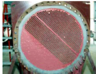
Tube sheet repair performed for Carrier Corporation.
